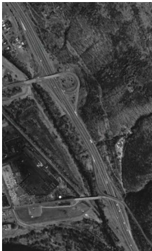
Image from Google Earth/U.S. Geological Survey (1994)
